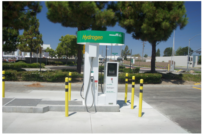
Figure 1. Hydrogen fueling station at the Orange County Sanitation District's municipal wastewater treatment facility in Fountain Valley, CA. Photo courtesy of Air Products and Chemicals, Inc.
