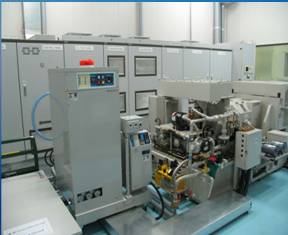
Motor Test Equipment (100 kW Class)
