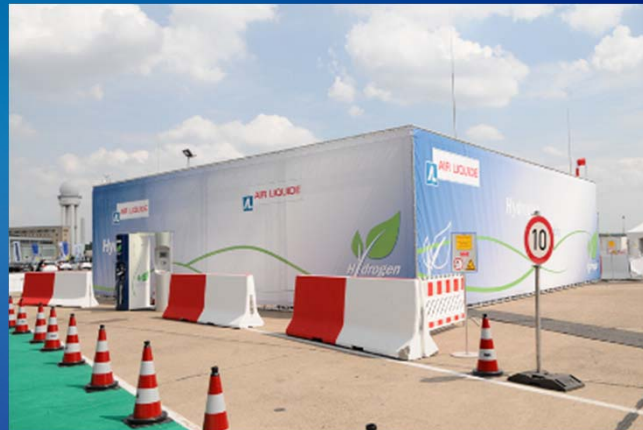
<Mobile H2 Fueling Station (700 bar)>
