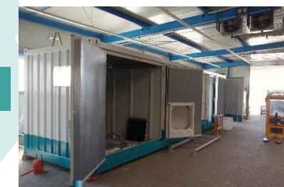
ReleaseBOX 10 (currently under construction)
