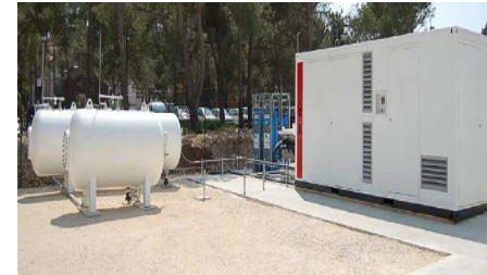
AREVA's energy storage platform 'GREENERGY BOX' in Corsica, France Utilizing Giner Low-Cost Electrolyzer Stack
