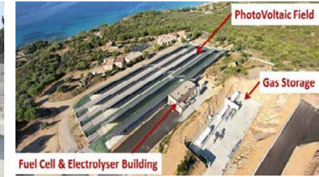
AREVA's energy storage platform 'GREENERGY BOX' in Corsica, France Utilizing Giner Low-Cost Electrolyzer Stack
