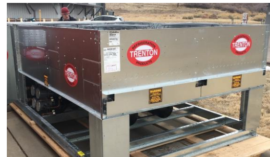
60 horsepower chiller at NREL's site
