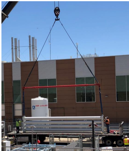
Crane lifting new high-pressure ground storage into place
