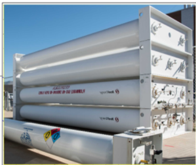
HYDROGEN STORAGE SYSTEM
