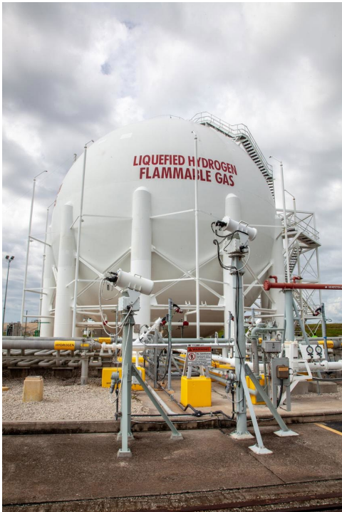
800,000 gal (3,3028 m 3 ) LH2 Tank at Pad 39B (NASA Image KSC-20191108- PH-JBS01_0001)
