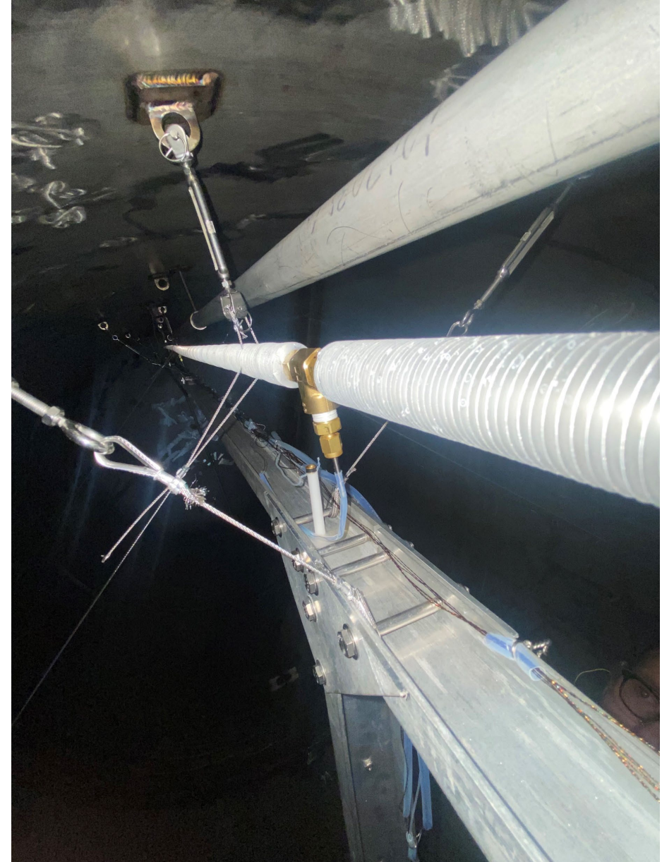
Image of HVT installed in tank.
