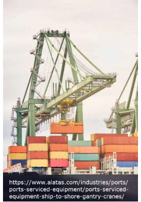
1x STS crane direct electric
