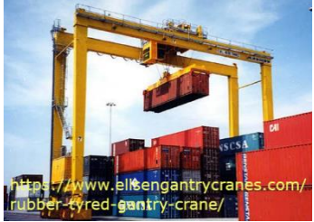
2x RTG crane direct electric
