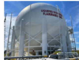
LH 2 storage tank 5,000 m 3
